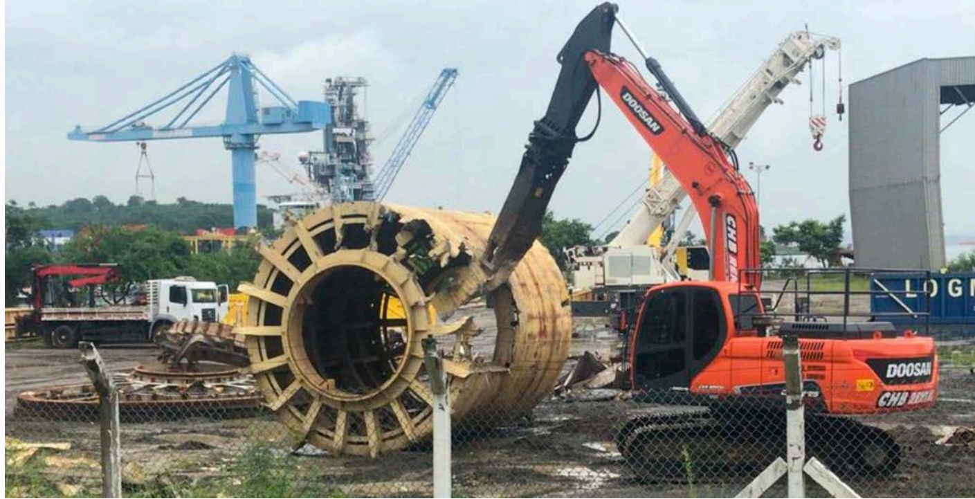
Decommissioning of coils and other components
